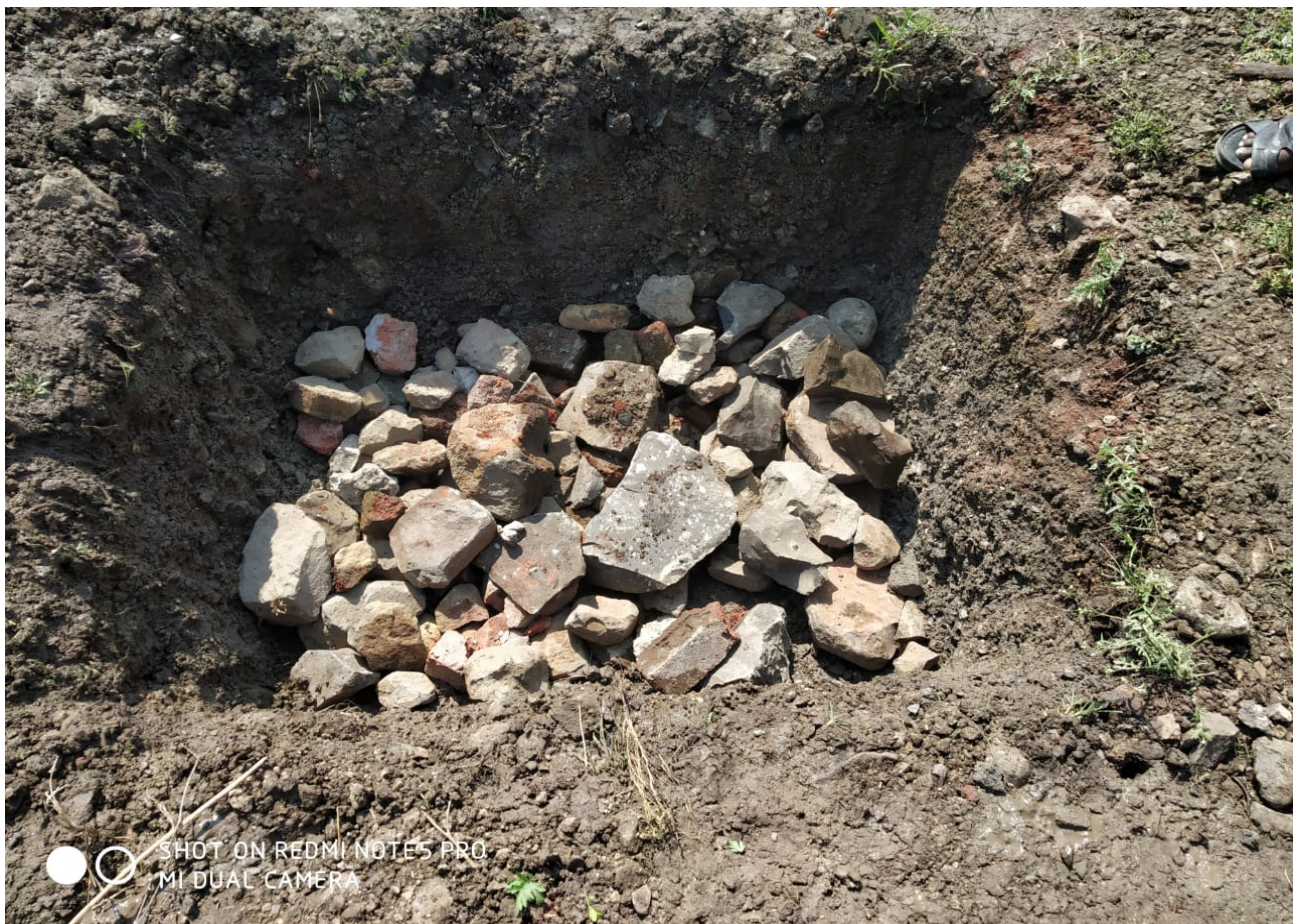
Student of NSS while constructing the suction pit
