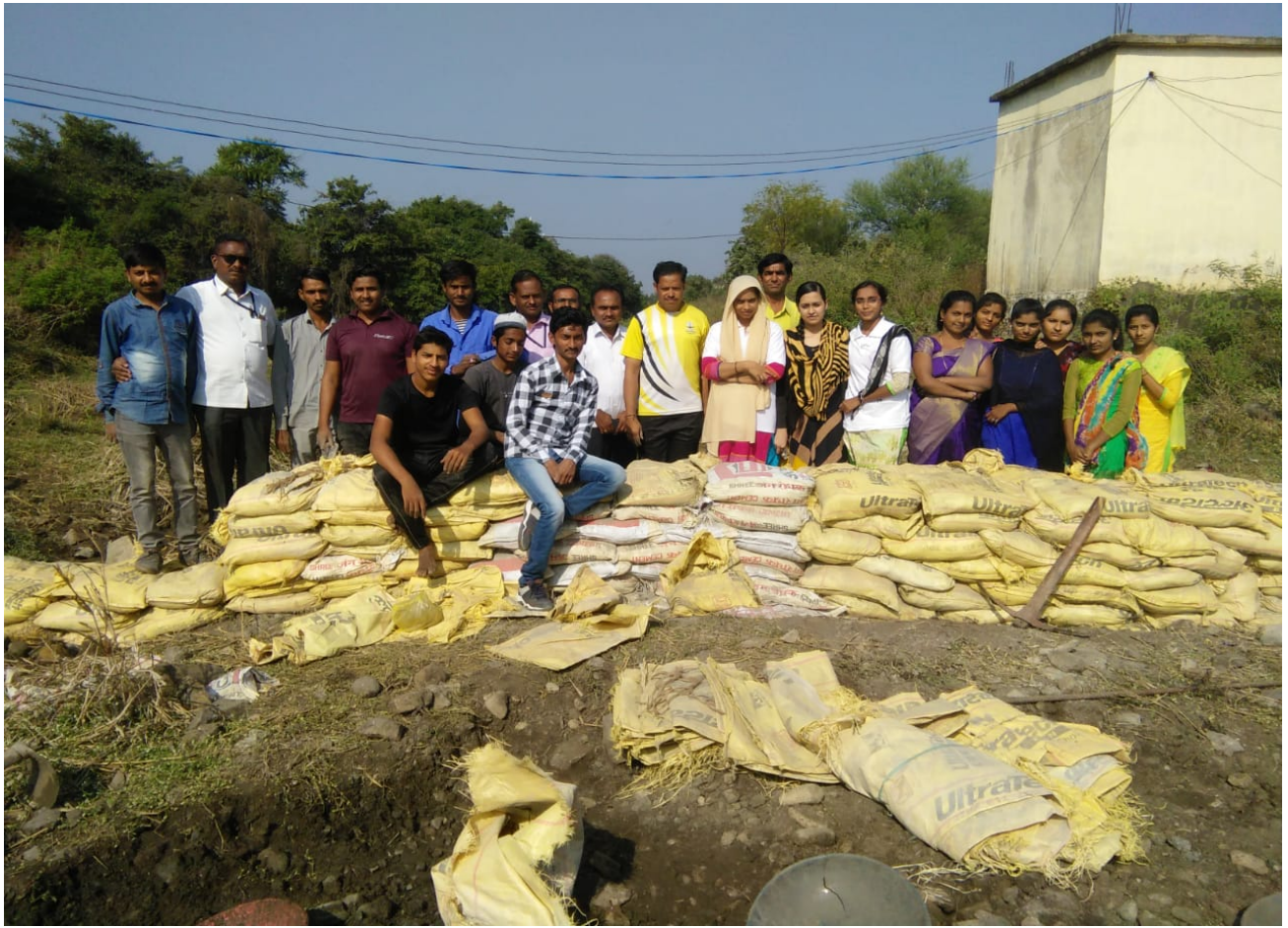
NSS students constructing the Cement sack dam
