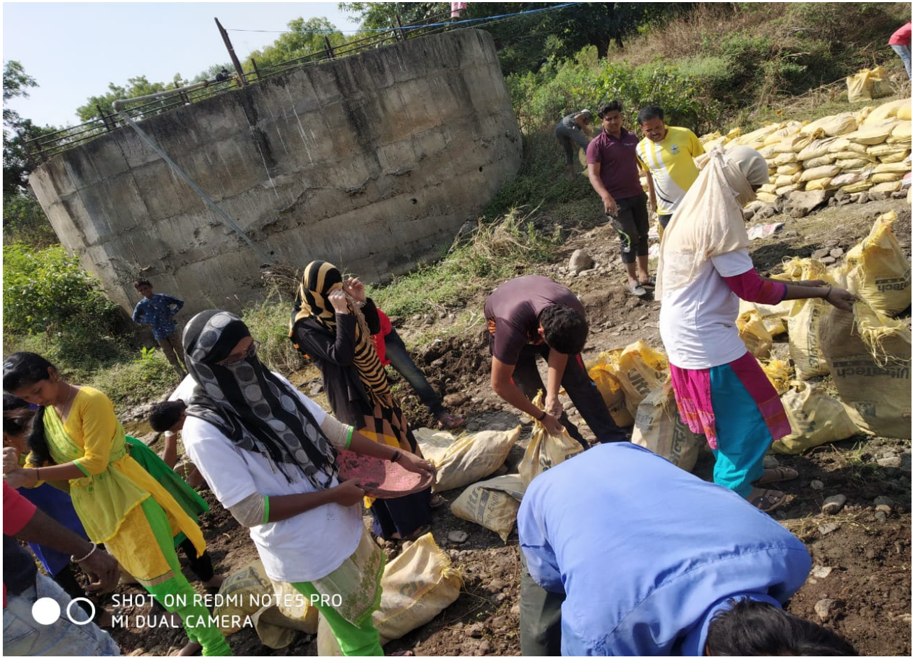
NSS students constructing the Cement sack dam
