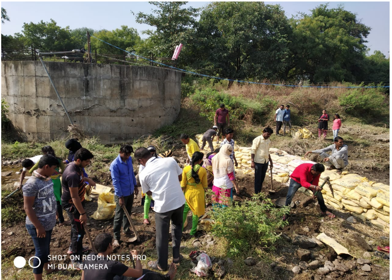
NSS students constructing the Cement sack dam
